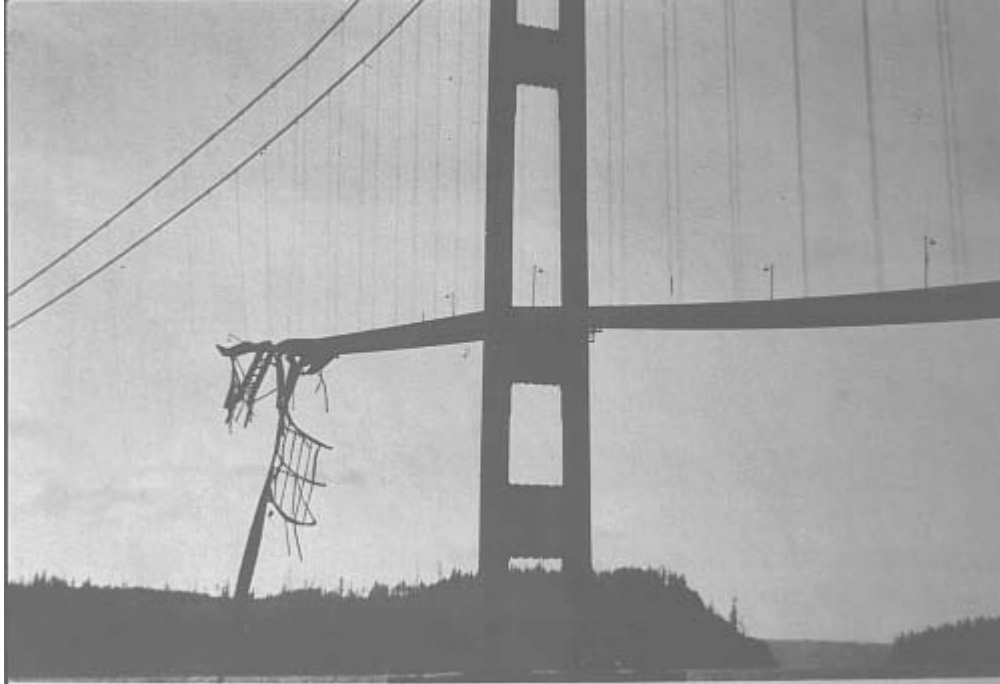
Figure 2b. Tacoma Narrows Bridge after the Failure
