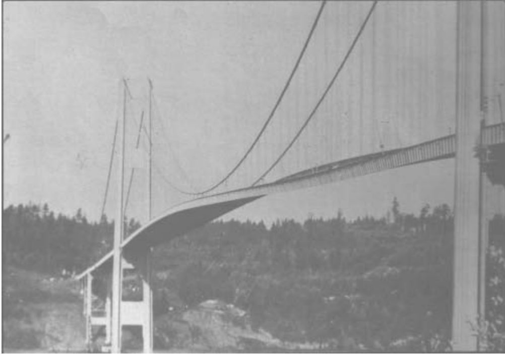
Figure 1a. Torsional Mode of the Tacoma Narrows Bridge
