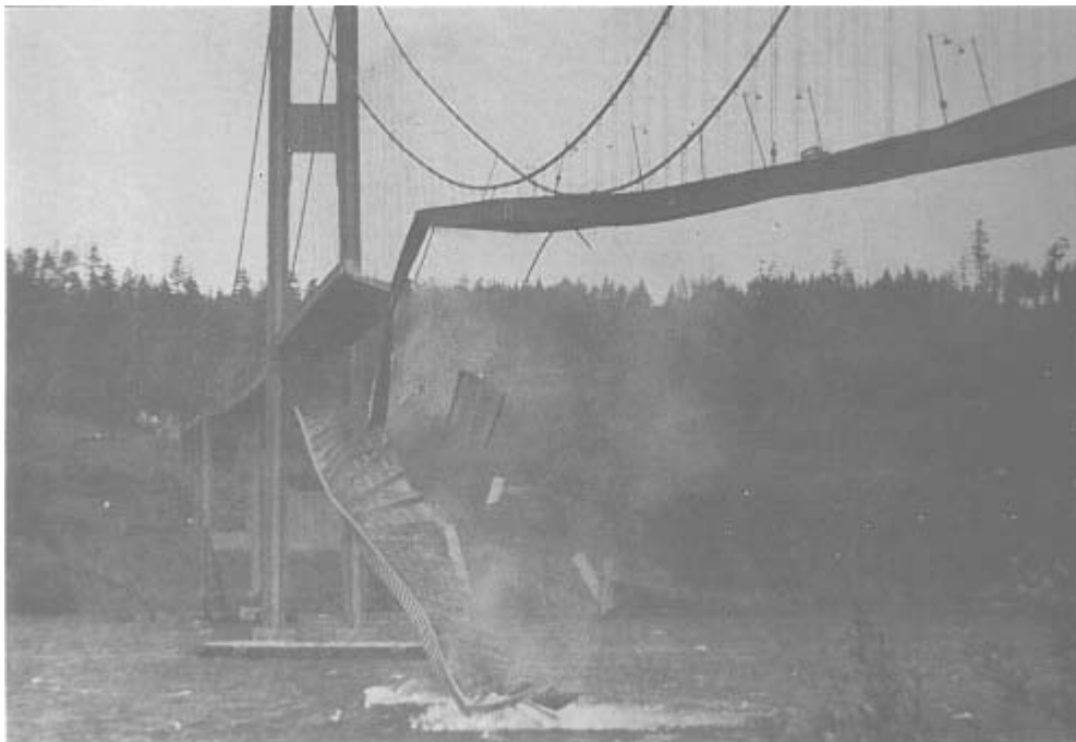
Figure 2a. Failure of the Tacoma Narrows Bridge
